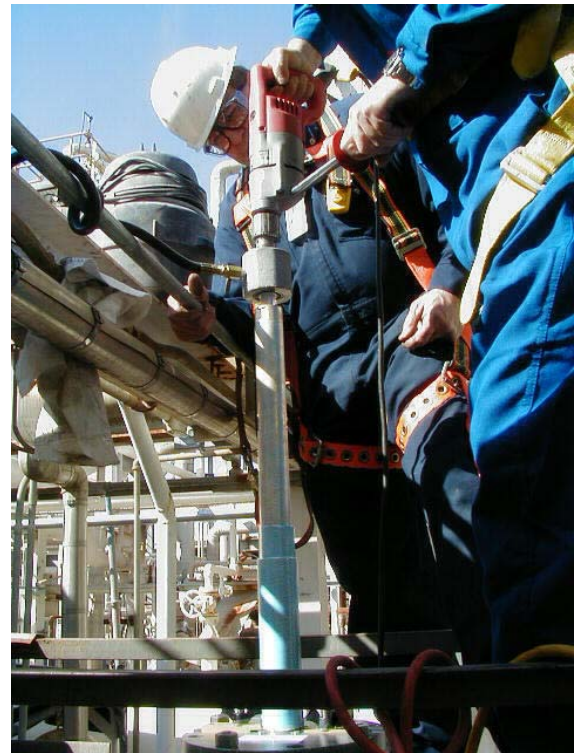
Hole Being Drilled Through Refractory In a Claus Thermal Reactor
