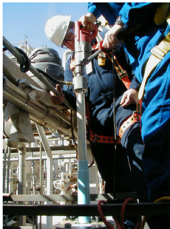
Hole Being Drilled Through Refractory In a Claus Thermal Reactor
