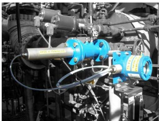
**Figure 10 Two-color pyrometer can provide early warning of occlusion before accuracy is compromised.**
