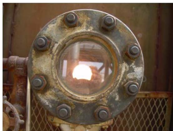
**Figure 2 Material collecting in the bottom of a sight port nozzle. Similar occlusions can occur in pyrometer process nozzles.**
